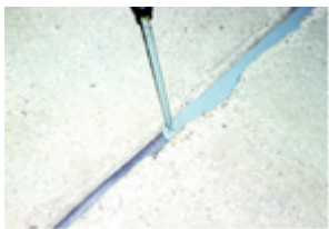
Compression, adhesion, and elongation determine successful control joint filling.
